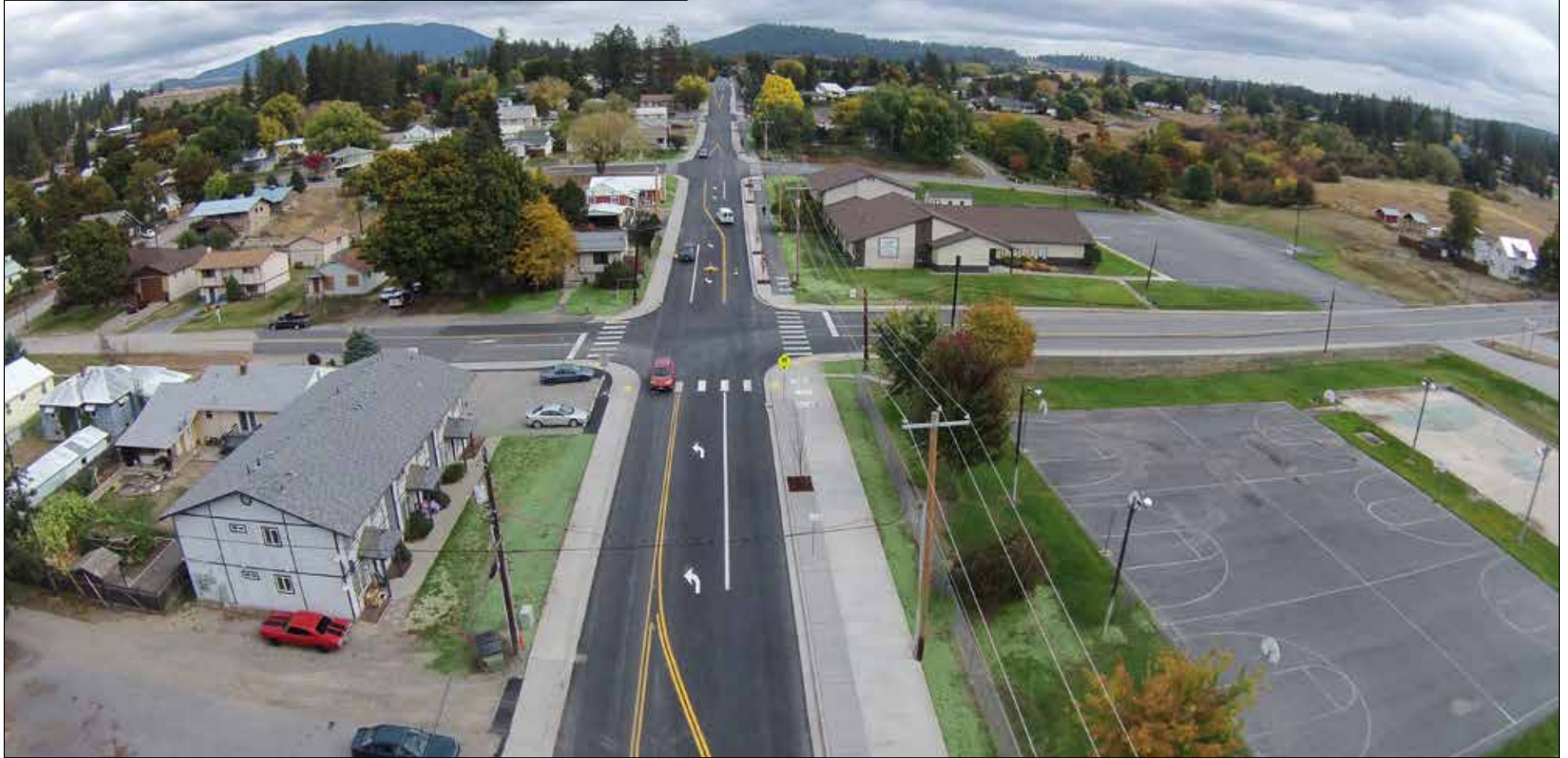
PHOTO COURTESY OF WELCH COMER ENGINEERS
