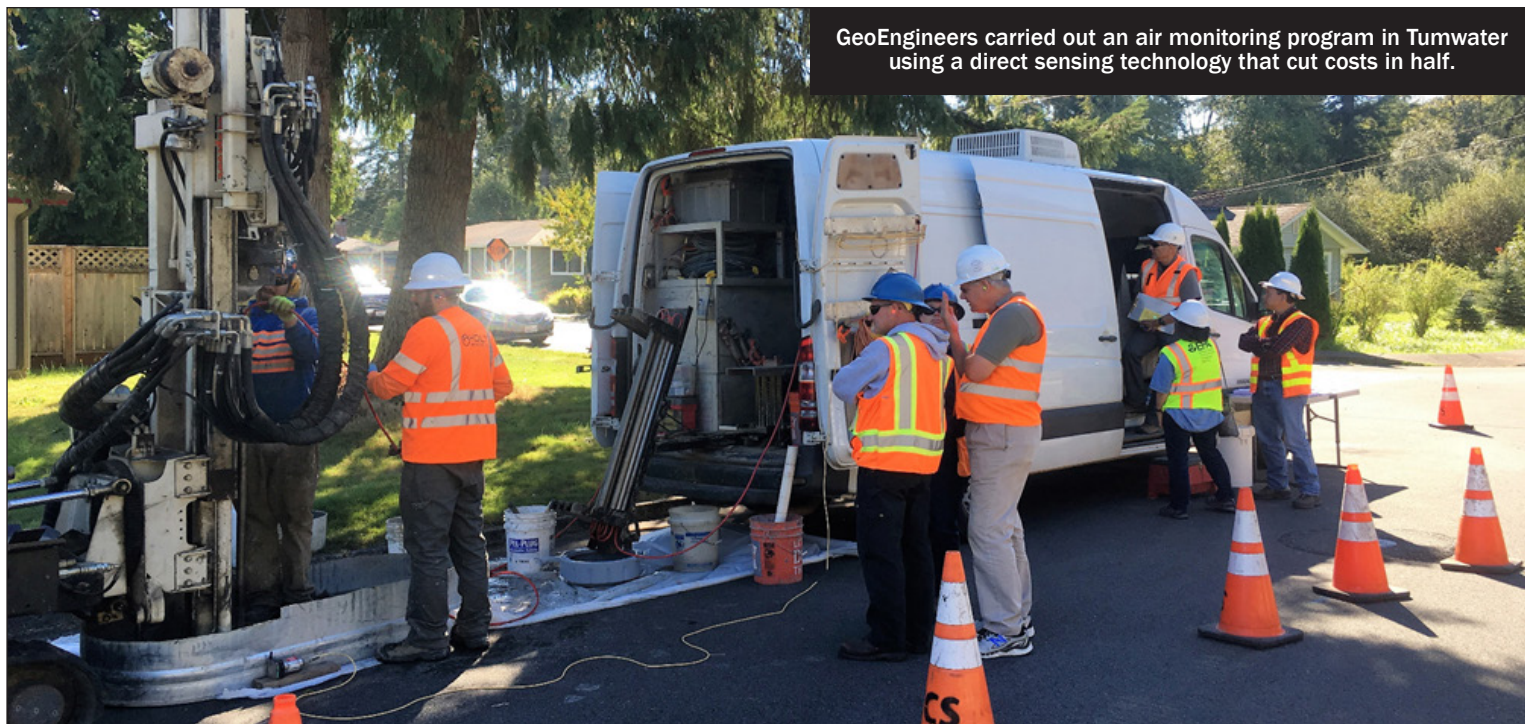
PHOTO PROVIDED BY GEOENGINEERS
