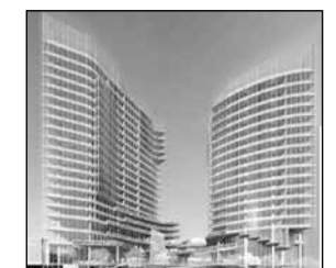
10 S O M A Phase II 10608 N.E. 2nd St. • 15,000 SF commercial • 124 units Developer: SU Development
