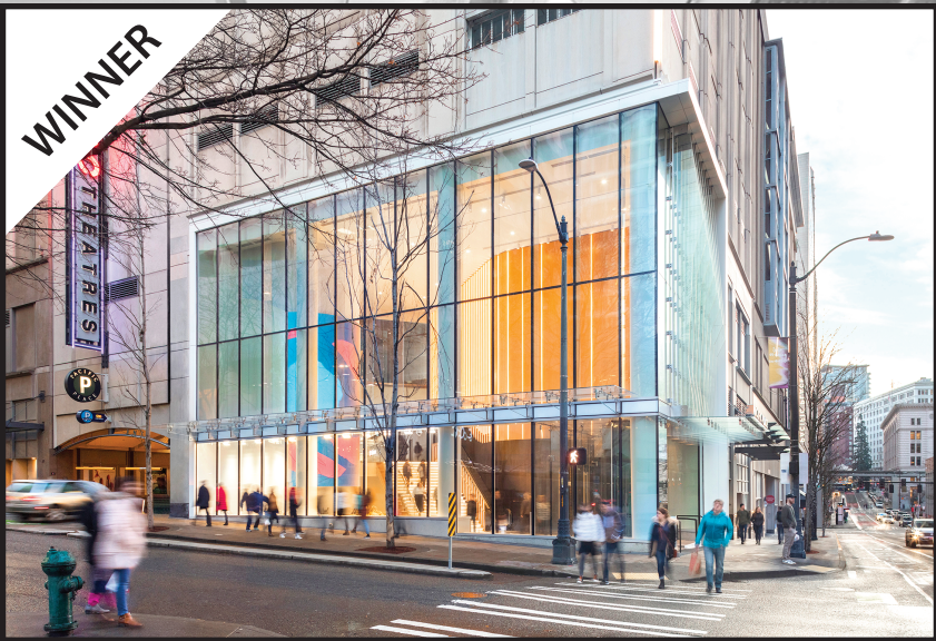
Private Building: $20M – $50M Pacific Place Retail Center | Seattle, WA
