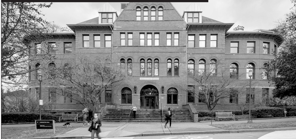
PHOTO FROM ABSHER CONSTRUCTION CO.
