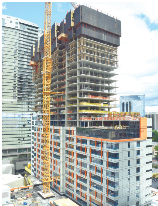
The W Hotel tower's innovations included the use of high-strength steel fiber reinforced concrete in the shear wall coupling beams, the largest use ever in North America.
