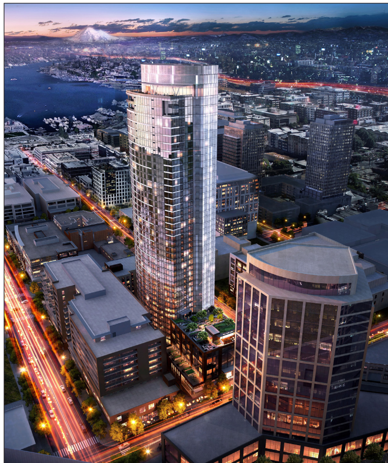
970 Denny, a residential high-rise under construction in South Lake Union, used early energy modeling to demonstrate that efficiency from the water source heat pump system would offset increased thermal loss from expansive glazing.
