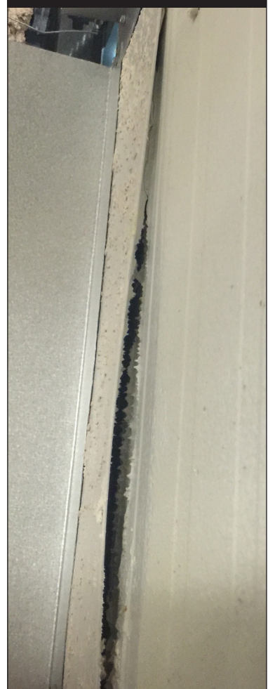
This sealant joint separated likely due to movement of the flashing.
