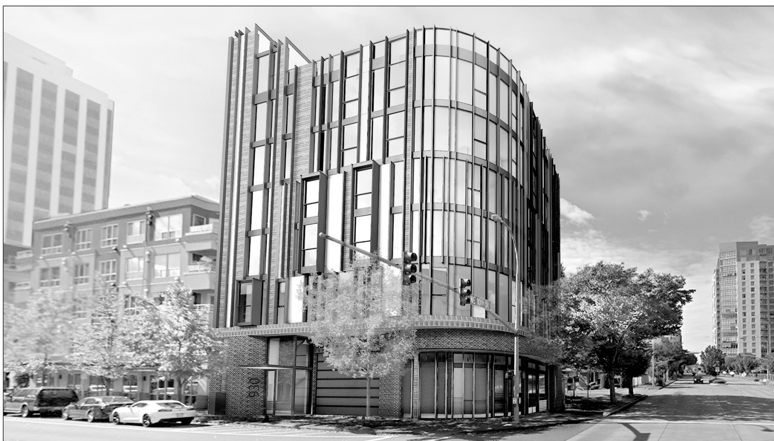
GIS Plaza is a six-story mixed-use building featuring 16 luxury condominiums, commercial space, and the first mechanical auto-valet stacked parking system of its kind in downtown Bellevue — all with sweeping views of lush-green parks, old-growth trees and other residential communities.
