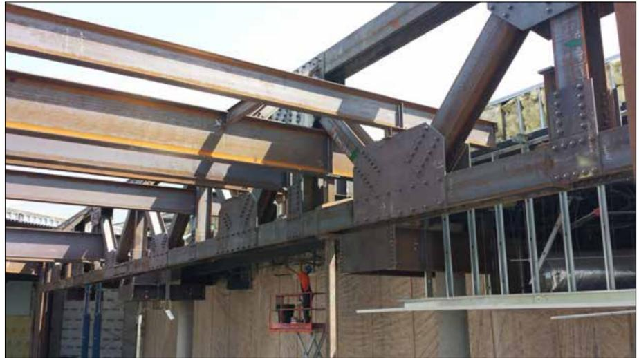
The expansion required 16 long-span trusses, which were pieced together on site.
