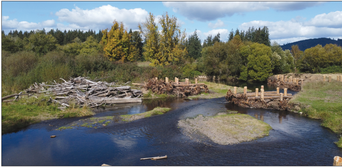
A large-scale river and floodplain restoration project on the Skookumchuck River at Riverbend Ranch in Thurston County restored more than 2.5 miles of river channel through the placement of engineered log jams.
