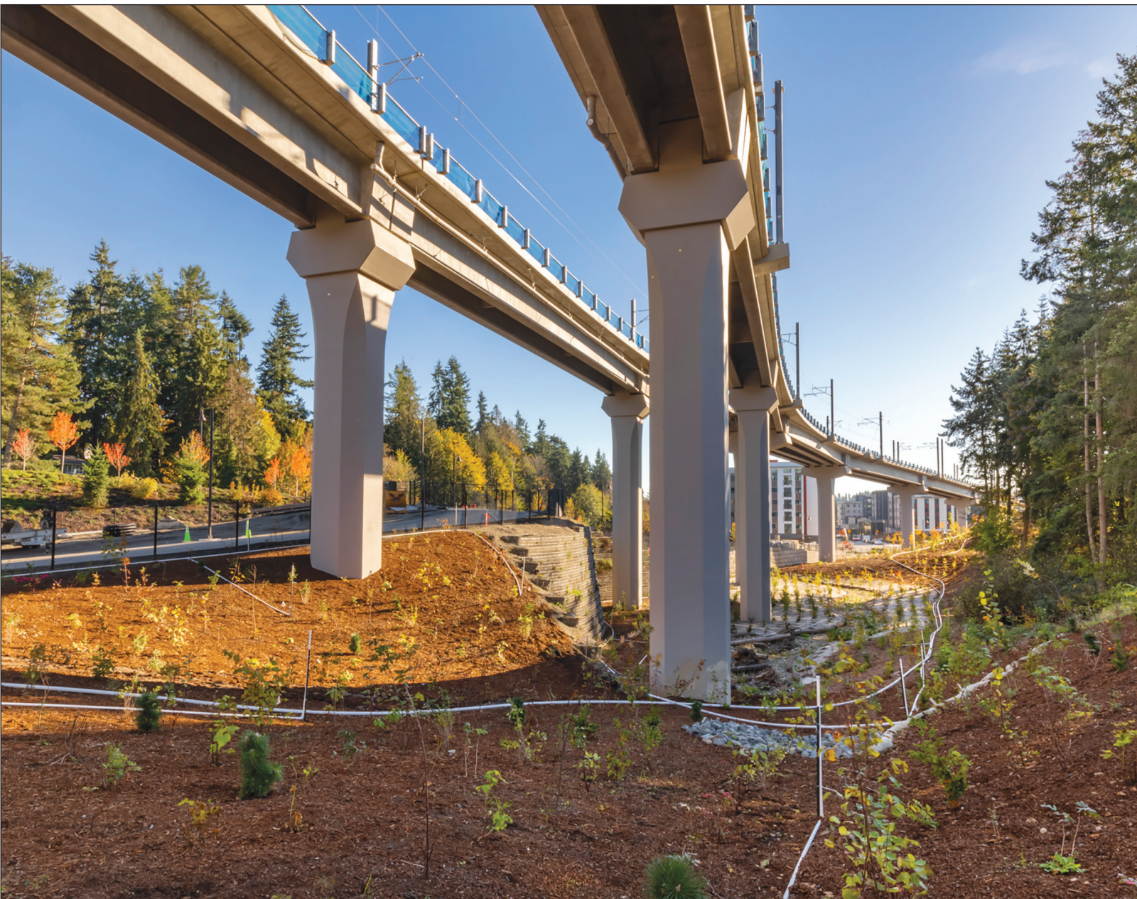
The recently completed L300 project included building 3.8 miles of aerial guideway, two elevated stations and a five-story parking garage at Lynnwood Transit Center.
