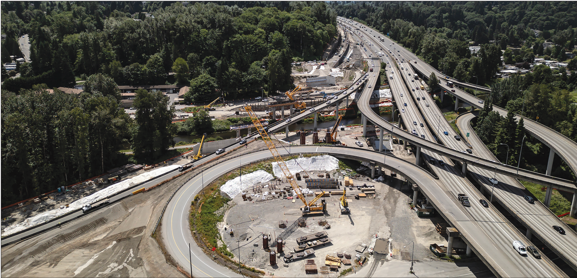
The Brickyard project will add the region's second, third and fourth in-line Bus Rapid Transit stations with direct access to express toll lanes.
