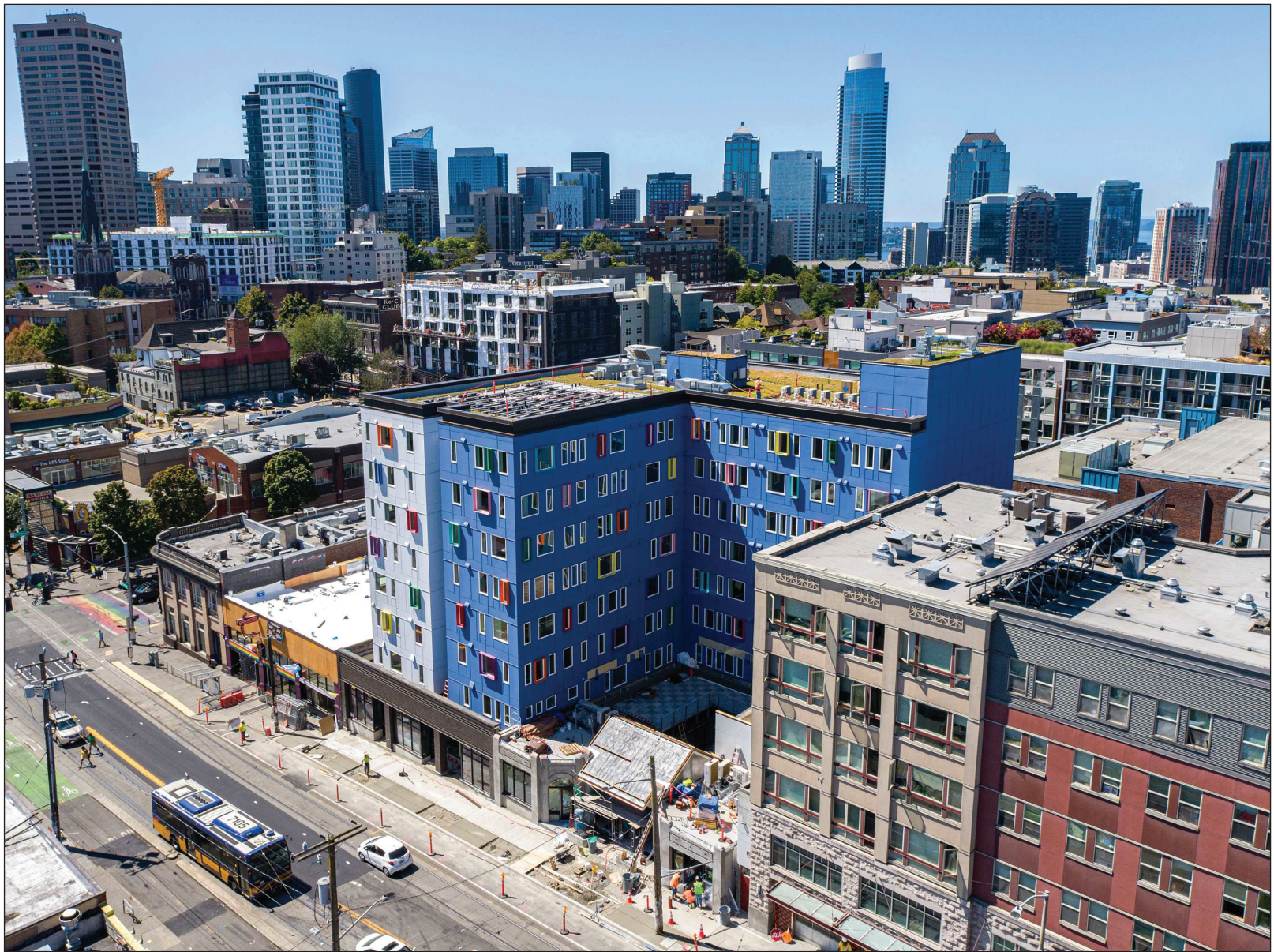
Walsh's project team was able to deliver the 118-unit Pride Place project to Community Roots Housing in late 2023 with zero safety incidents. Photo by NW Skyview Imagery
