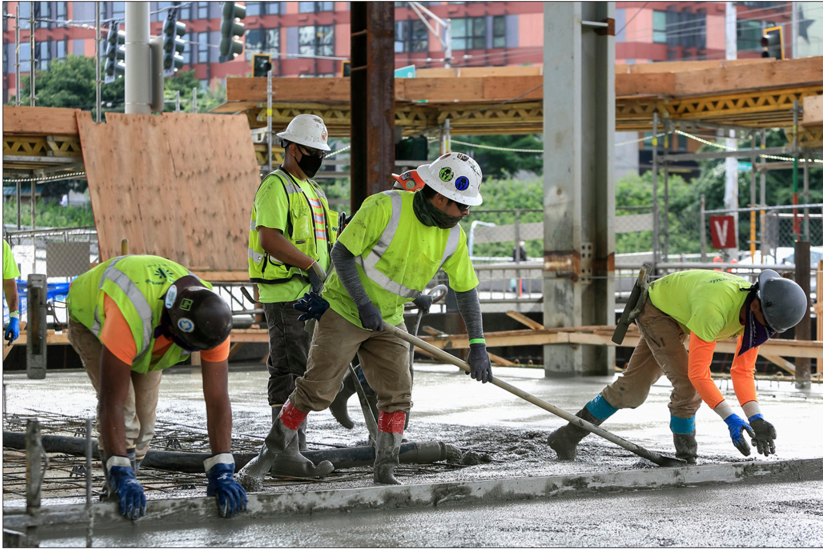
A concrete crew completes a pour at the Summit building.
