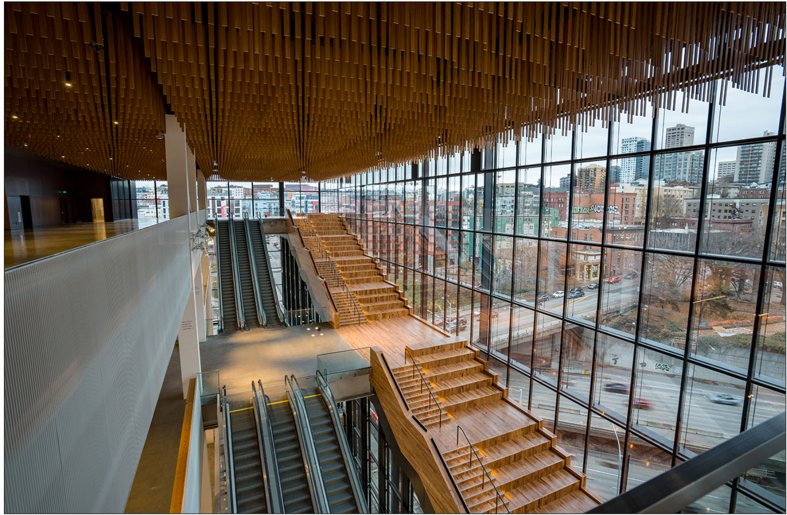
Radiant floors extend into the wooden hillclimb seating stairs.
