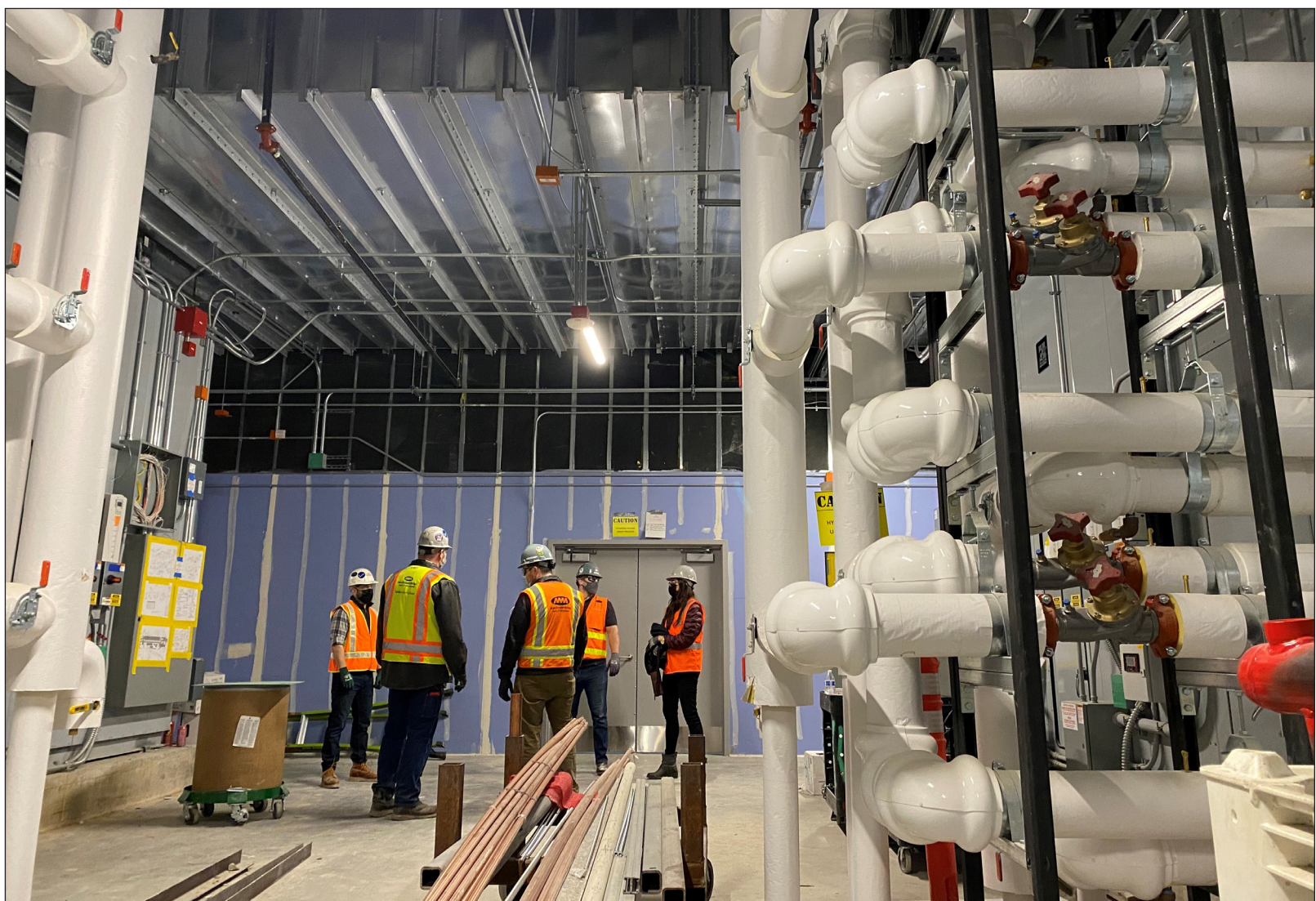
Dual-temperature air-handling unit coil connections, in the foreground, supply the air header in the background.
