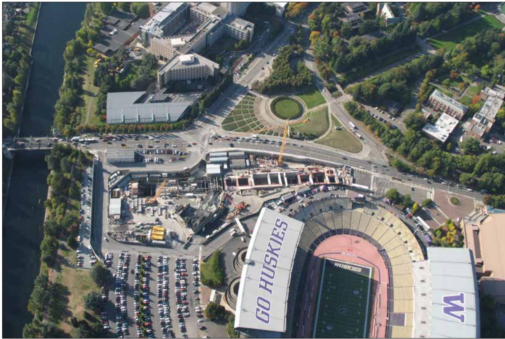
The tunnel crosses under Montlake Cut by Husky Stadium.
