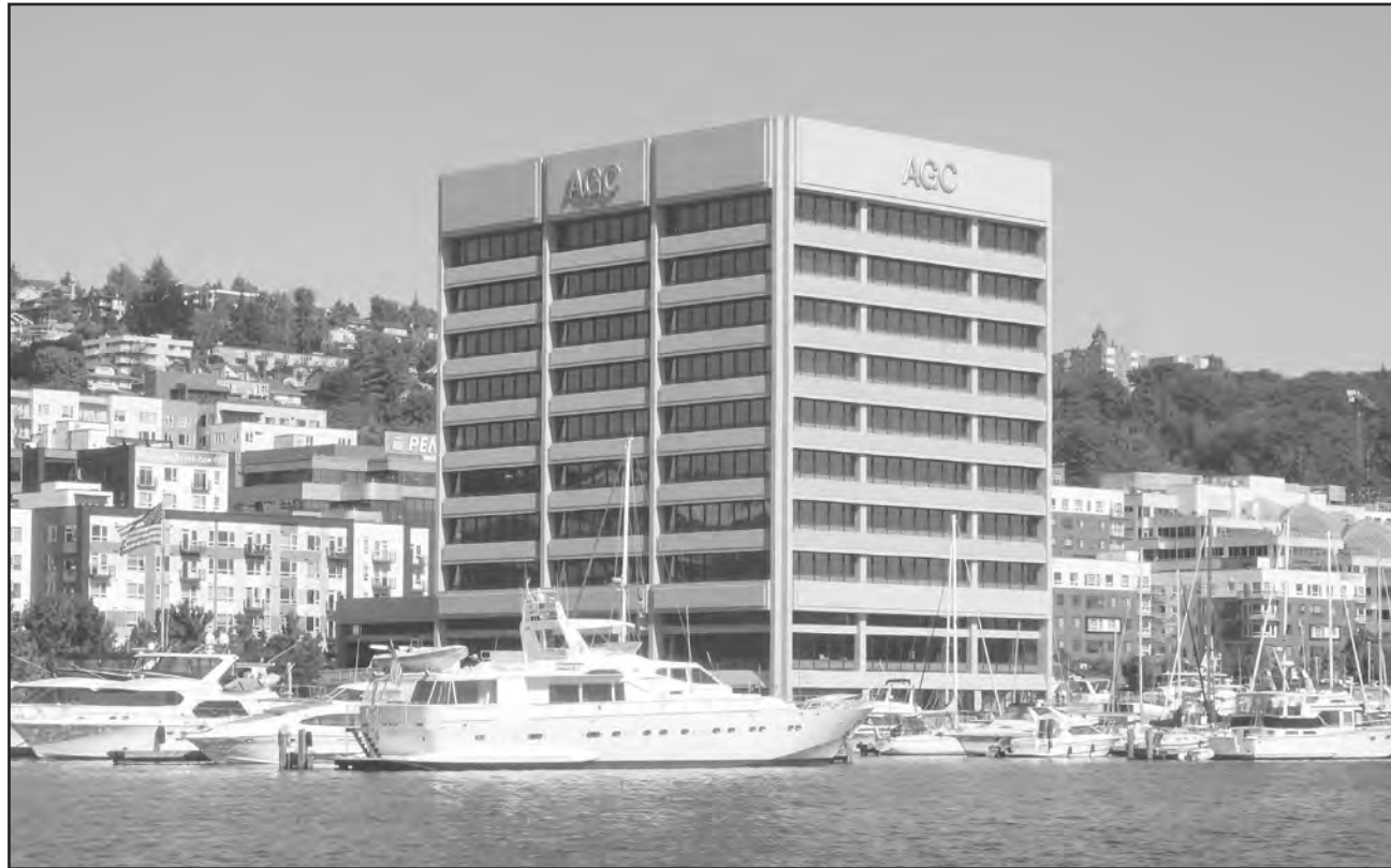
The ten-story, 114,789 s.f Seattle AGC Building was constructed in 1971 on the southwest shores of Lake Union.
